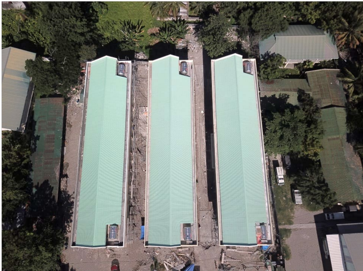
Sample arrangement of school buildings arranged in rows following the suggested orientation.
