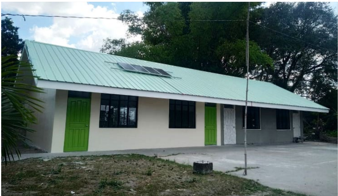
Prototype of LMS Building Using Light Materials constructed in Mabalacat Elementary School in Pampanga
