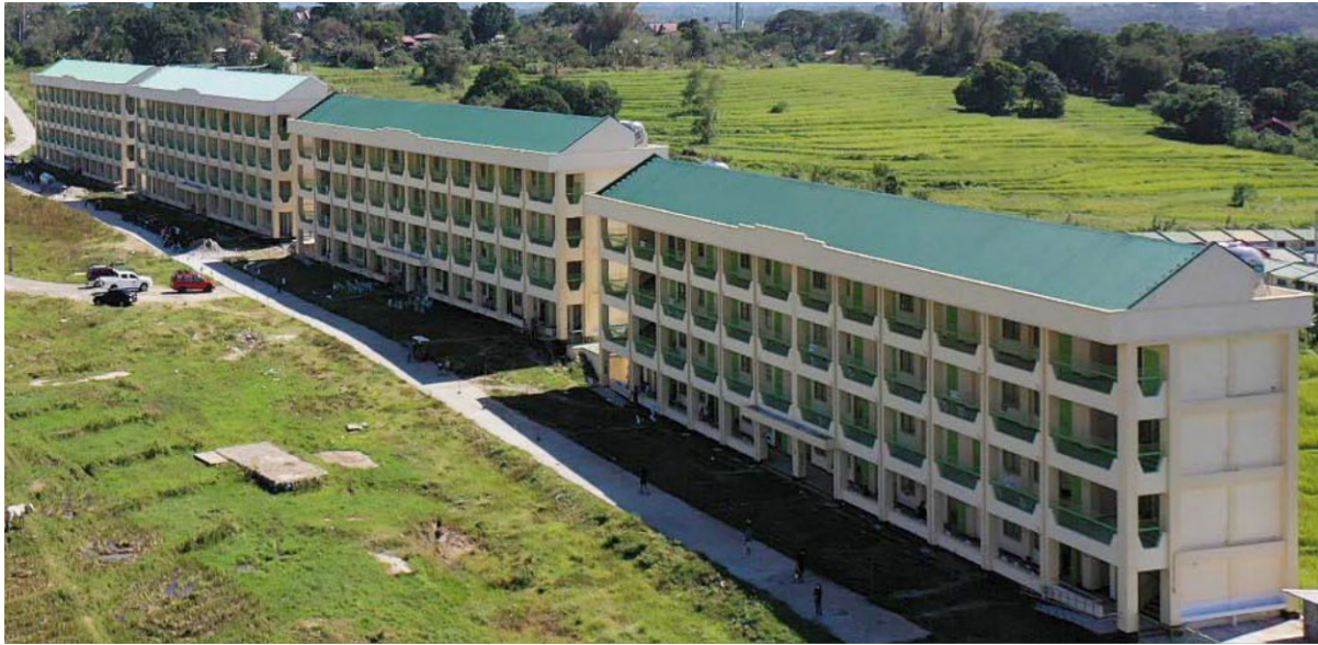
Sample arrangement of school buildings arranged along the perimeter line of the school property to maximize the open area at the center of the property for school activities.
